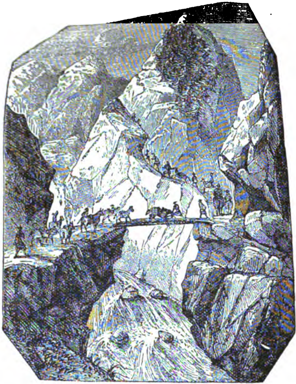
Bridge of Ghamda.
